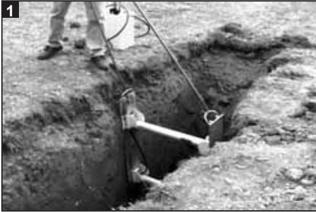
1 To remove the shore, place the removal tool through the handle with the hook facing the trench. Place the end of the tool over the same fitting where hose was hooked.
