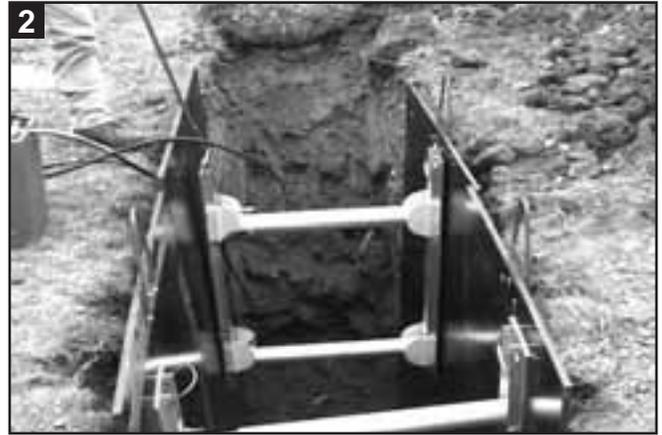
2 Release the top rail and allow shore to completely unfold. The shore will lock itself into open position.
