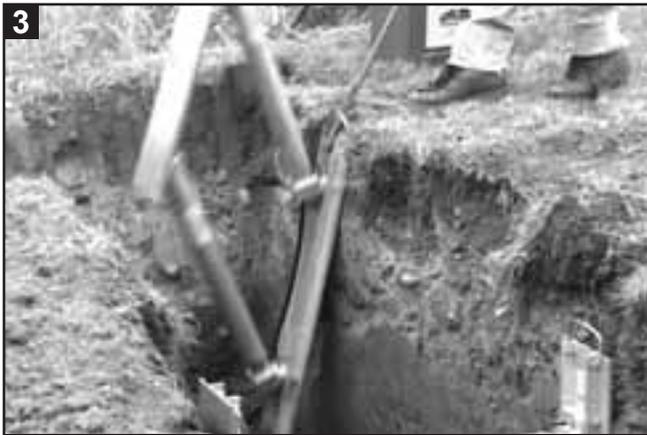
3 Remove from trench by pulling one side with release tool and the other side with the removal hook.
