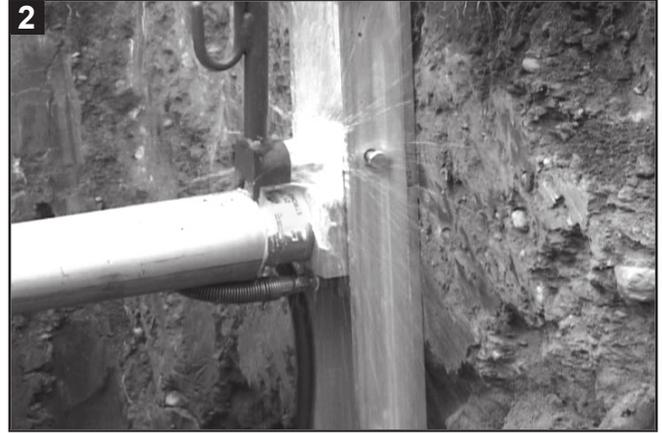
2 Push the tool away from you against the handle. The tool will depress the fitting and release a small amount of fluid.
