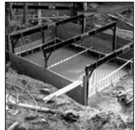
Large, three-sided configuration with hi-clearance arches and splice plates
