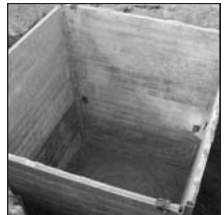
Two, 8x8x8 ft. stacked Build-A-Box with Stacking Guide accessory
