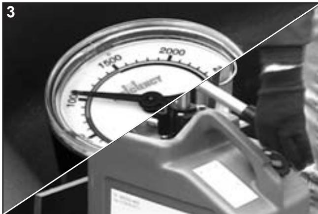
3 While holding the shore at the desired height, close the 1/4 turn release valve on pump can and pump the handle on the can to build pressure between 750-1500 PSI.
