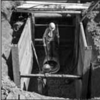
Two-sided configuration with telescoping spreaders and full length corner posts
