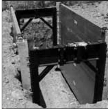
Two-sided configuration with full length corner posts and arches
