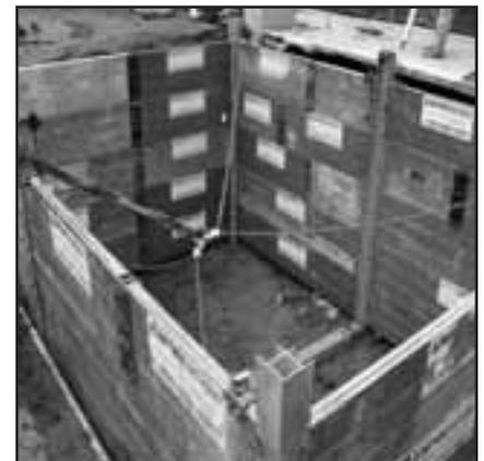
ClearSpan™ Configuration with full length corner posts
